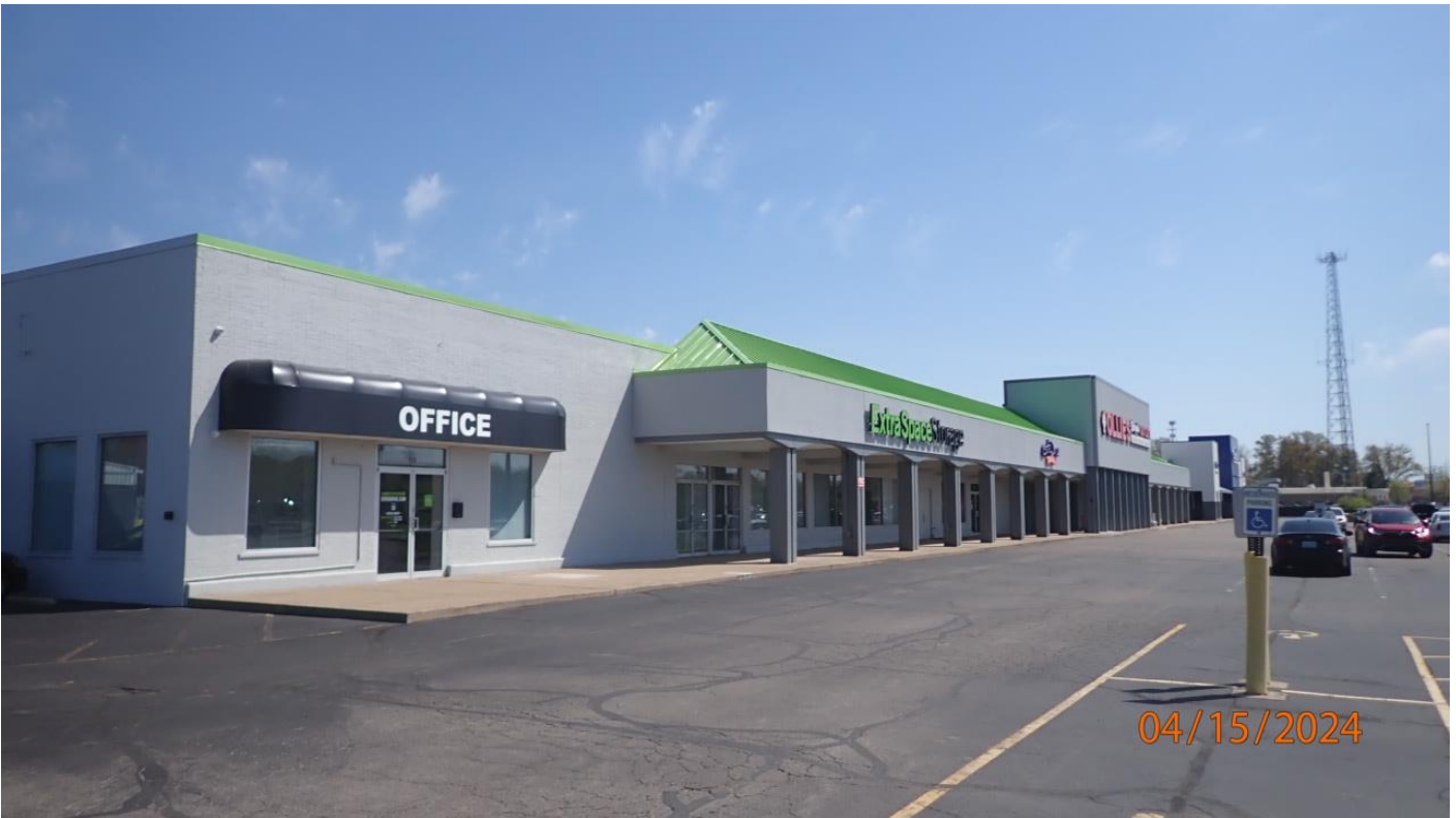
View looking northeast from parking lot.
